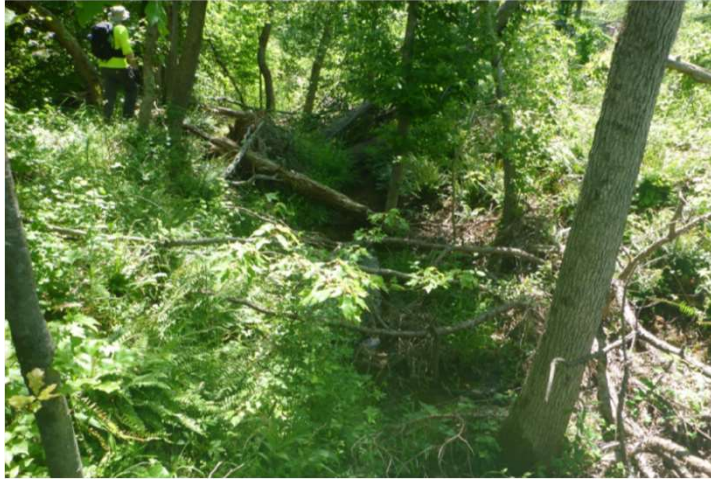
Remarks: UT 2 - Upstream View (Facing East)
